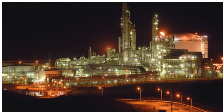
FIGURE 11.3.3 The Yara Pilbara Fertilisers ammonia plant in Western Australia is one of the world's largest ammonia plants, with an annual production capacity of approximately 850 000 tonnes.
